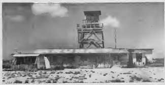
No, it isn't a toothed or a chicken coop, it's the old airport building, Aruba's first air-link with the outside.
